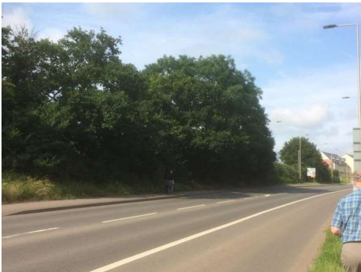
Hedgerow H1, London Road frontage to be removed to accommodate proposed roundabout junction into application site
